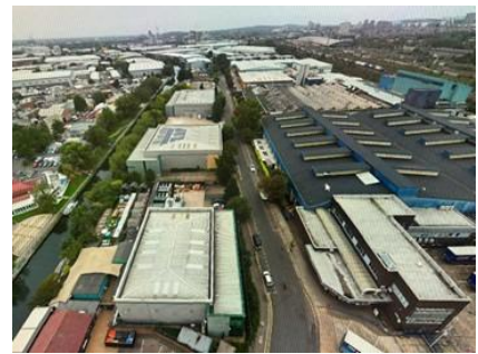
Figure 1. Roof area in food manufacturing facilities at Park Royal
