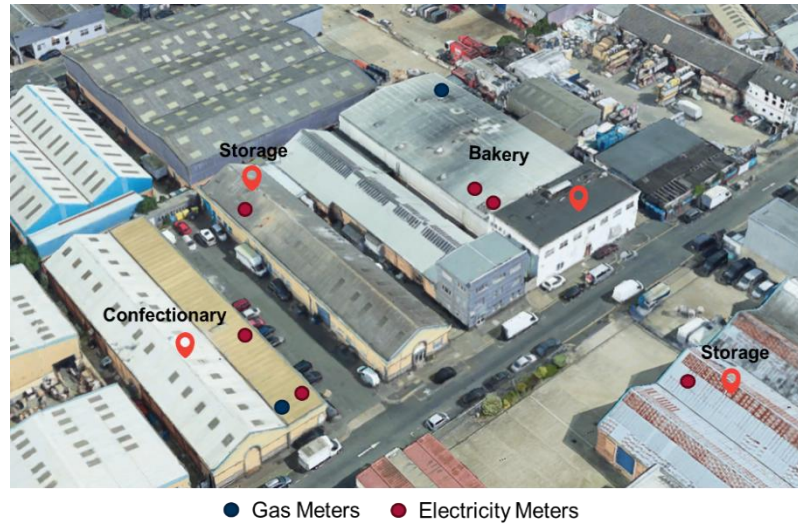
Figure 2. Confectionery manufacturing facility
